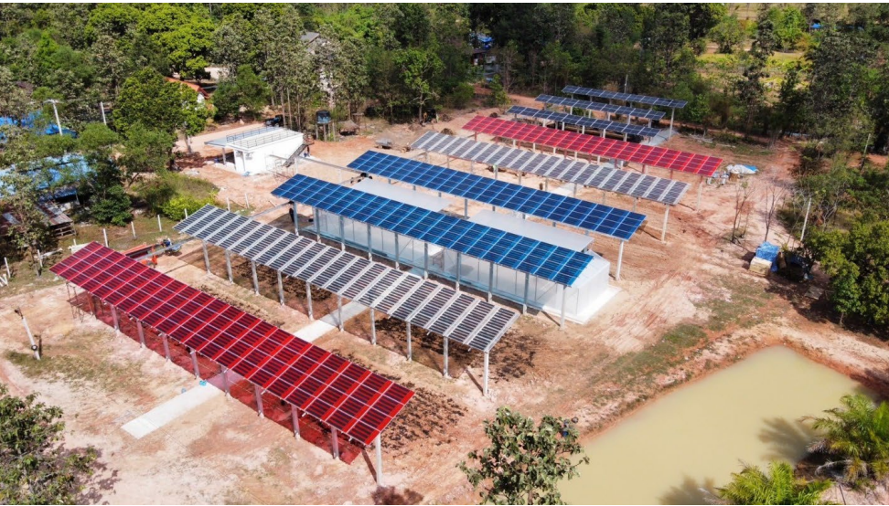
Figure 2.11 Colored PV system at Wat Pa Sri Sengtham, Khong Chiam District, Ubon Ratchathani Province.
