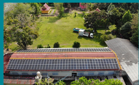
Figure 5.11 Microgrid PV system for sustainable community on Koh Jik Island, Chanthaburi province.
