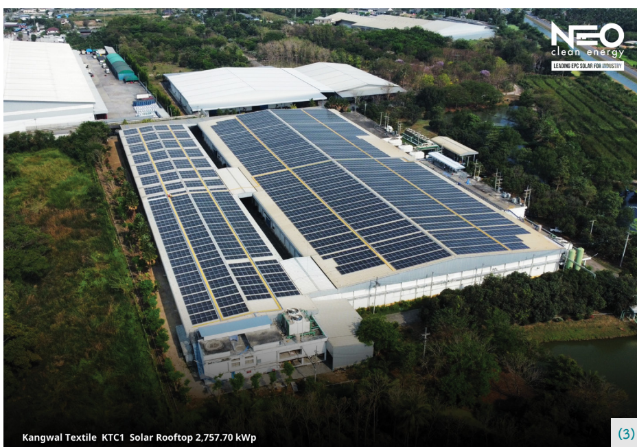
(3) 2.7 MWp rooftop PV system in Photharam, Ratchaburi province.
