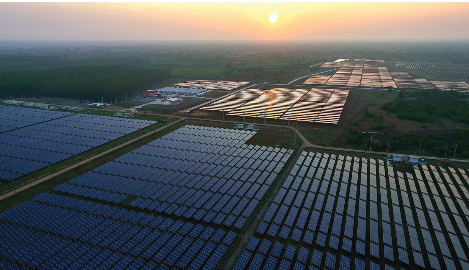
Figure 5. 4 Typical PV system with a battery energy storage system (BESS) and biogas power generation system installed capacity of 48.91 MWp, located in Han Sai, Aranyaprathet district, Sa Kaeo province.
