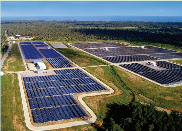
Thap Sakae PV power plant at Thap Sakae district, Prachuap Khiri Khan Province
